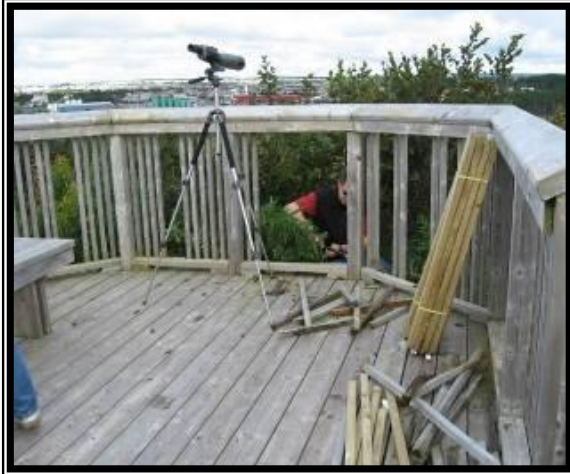
Fig 4. Vandalized Viewing Platform
