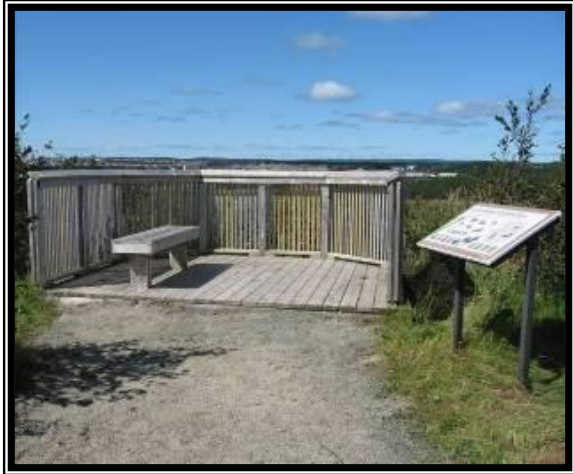
Fig 5. Repaired Viewing Platform
